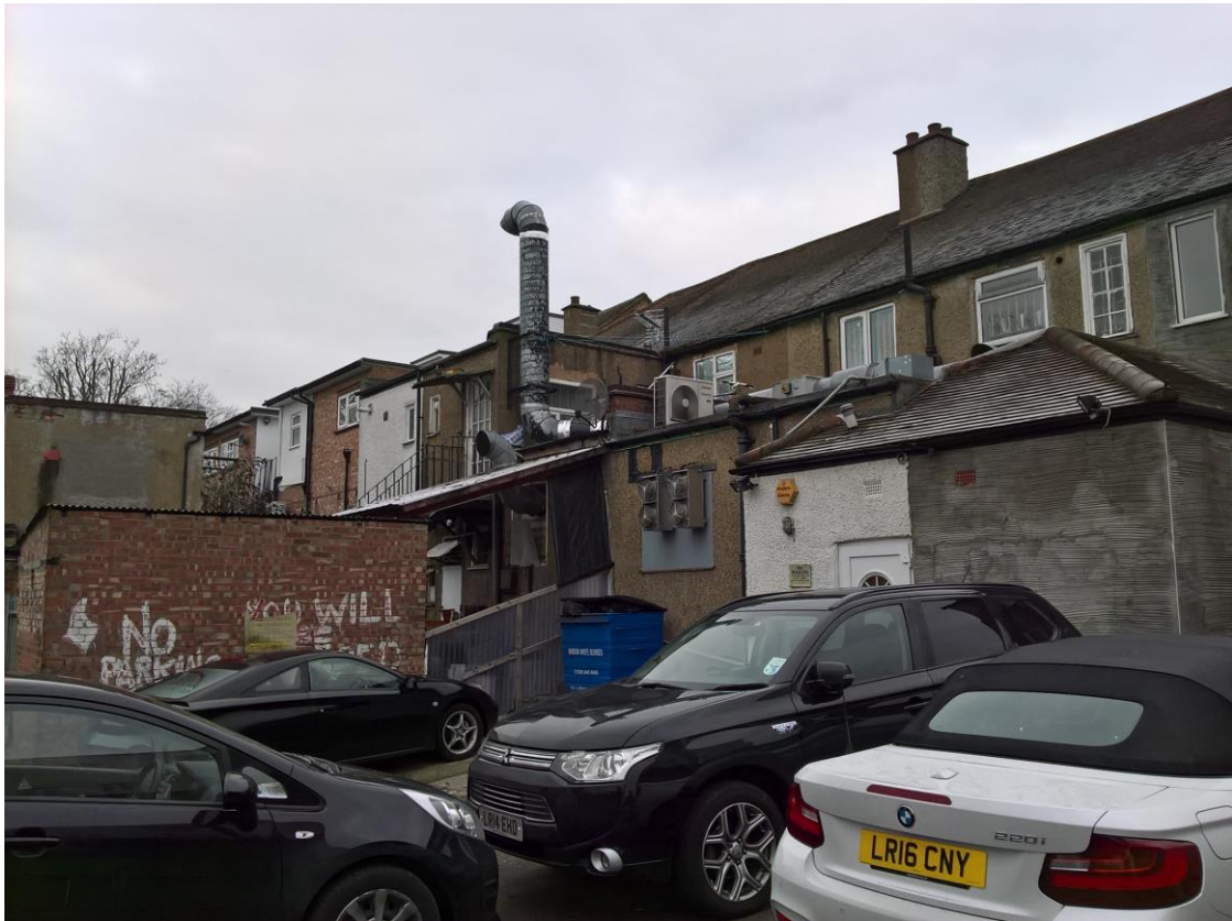
Rear of shops/flats to north on Church Road
